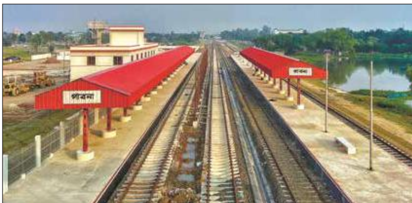
Newly constructed Pabna Railway Station under “Construction of a New Railway Line from Ishurdi to Dhalarchar Via Pabna” project.
