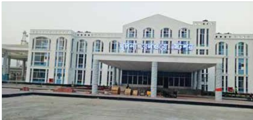
Newly constructed Khulna Railway Station Building under “Remodeling of Khulna Railway Station & Yard and Development of Operational Facilities of Benapole Railway Station” project.
